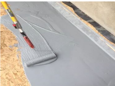
Surface Waterproofing
