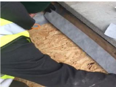
Waterproofing of Critical Areas
