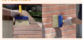
Ducky is based on silanes and siloxanes which form a water-repellent matrix within the masonry. With a low molecular weight **Ducky penetrate deeply** into the
