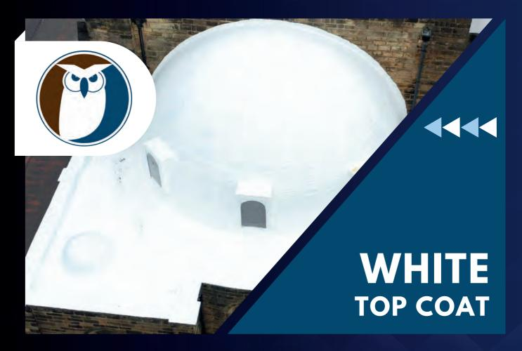
Enhance the aesthetic appeal of your surfaces with the Lava 20 White Top Coat, specially designed for application over the main Lava 20 Liquid Rubber Waterproofing Membrane. This one-component, deeppenetrating solution offers a decorative and color-stable finish.
